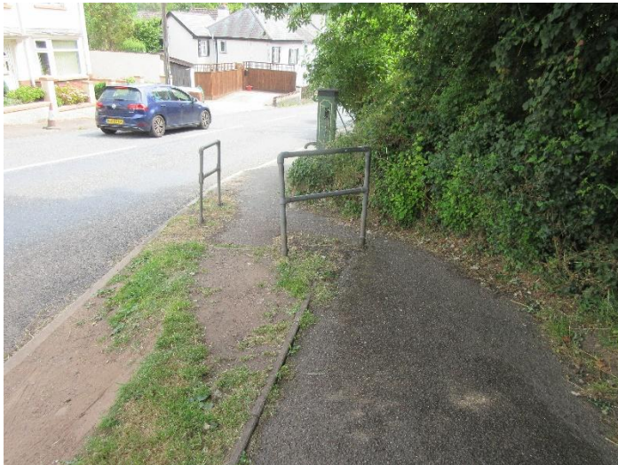
Steep gradient with narrow residual width of path
